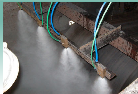
“Dry Fog” being added to coal over a conveyor head drum
